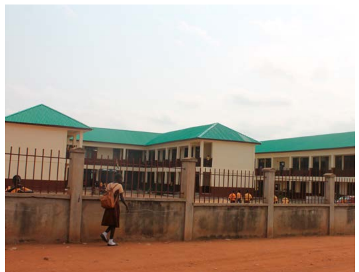
The newly built Ashaiman No. 2 Basic School block.
